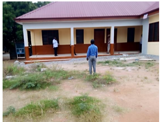
CONSTRUCTION OF 2 UNIT CLASSROOM BLOCK AT BORTIANOR
