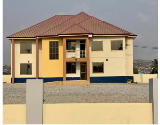
CONSTRUCTION OF POLICE DIVISIONAL HEADQUARTERS AT TUBA
