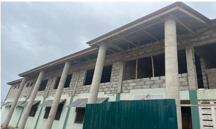
CONSTRUCTION OF UPPER FLOOR OF MOTHER AND CHILD WARD
