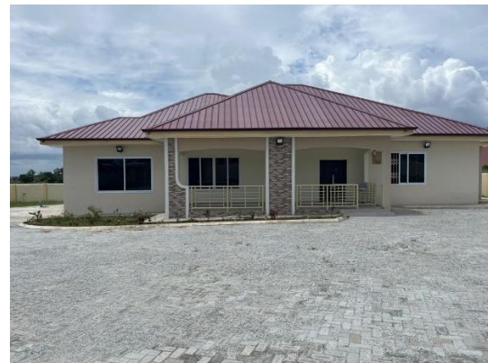
CONSTRUCTION OF MCE'S BUNGALOW AT TUBA
