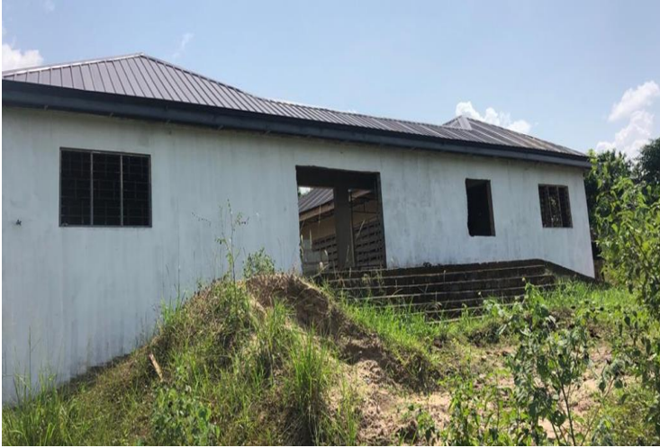
CONSTRUCTION OF CHPS COMPOUND AT FANKYENKO
