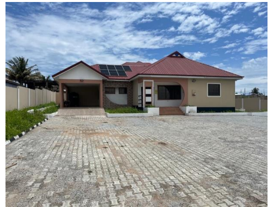
CONSTRUCTION OF COURT MAGISTRATES BUNGALOW AT TUBA
