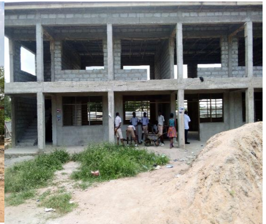
CONSTRUCTION OF SIX UNIT CLASSROOM BLOCK AT ASHALAJA
