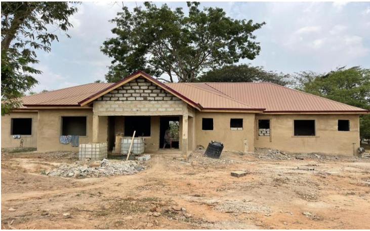
CONSTRUCTION OF MOTHER AND CHILD BLOCK AT OBOM
