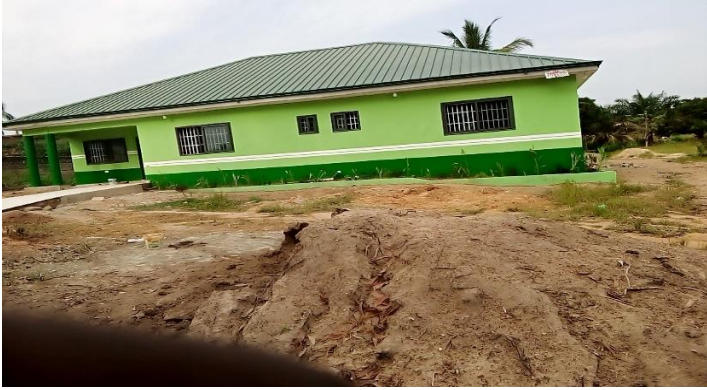
CONSTRUCTION OF 5-BED MATERNITY BLOCK AT KOKROBITE
