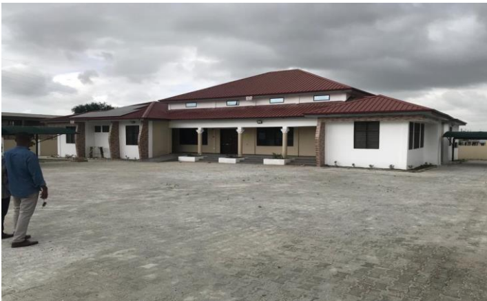
CONSTRUCTION OF MUNICIPAL COURT AT AMANFRO
