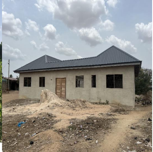
CONSTRUCTION OF CHPS COMPOUND AT DOMEABRA
